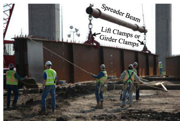
Fig. 1. Lifting of a curved I-girder with a spreader beam and lift clamps
